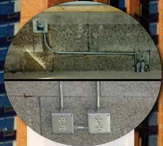
Accommodates electrical wires and services, either on or within the Nexcem surface
