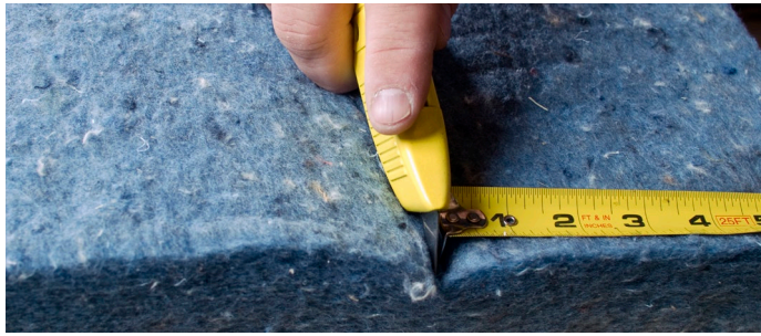
Measure and cut with a simple utility knife along Cotton Armor's width. A custom fit is yours with ease.
